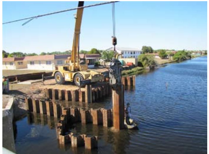
Worker Guiding Form Into Place - Oakland Hills Weir
