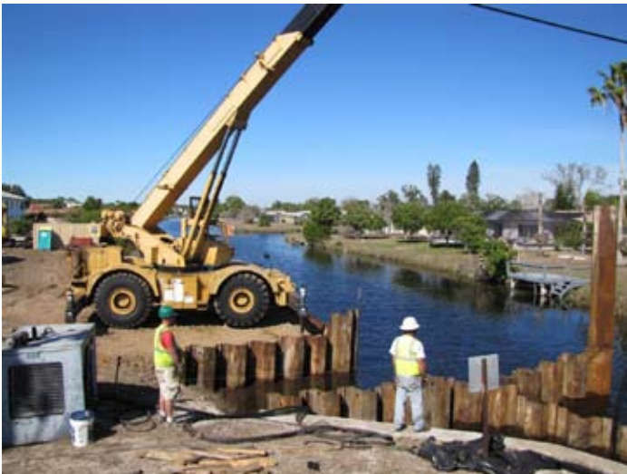
Workers Lowering Form Into Water - Oakland Hills Weir
