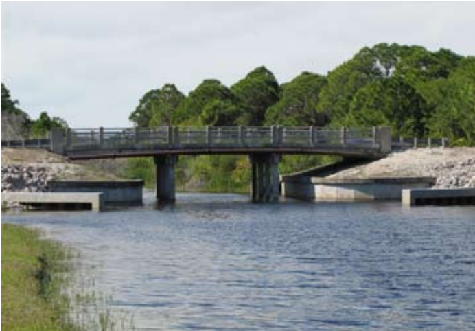
Completed Weir - Pine Valley - Ground View
