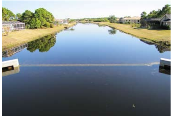
Completed Weir - Pine Valley - From Top of Bridge
